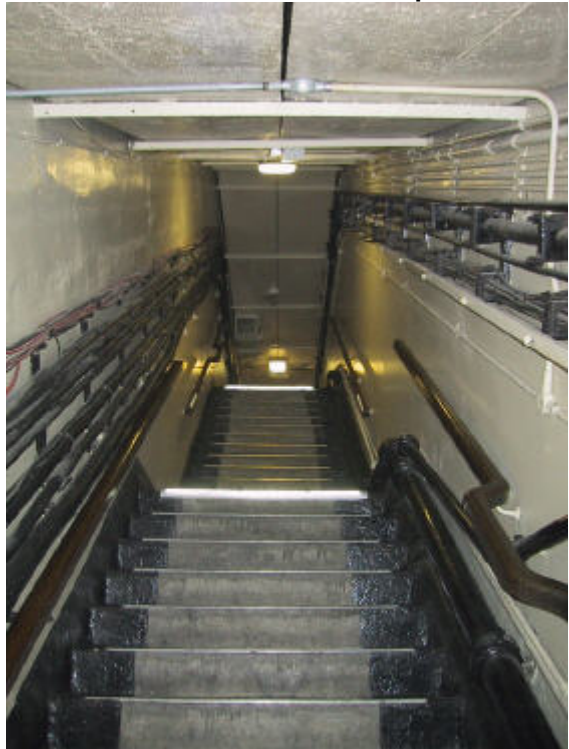
Looking back up the stairs to the outside world
